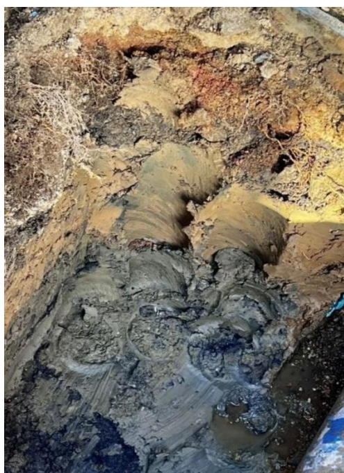
Figure 9.1 – Examples of poor excavating practices
