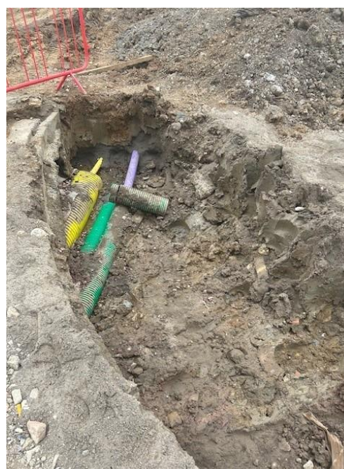
Figure 9.1 – Examples of poor excavating practices
